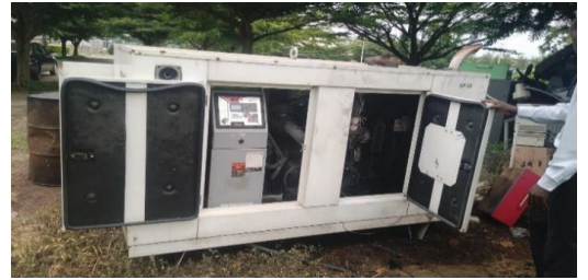
Fig. 5. Mikano SP 60 generator installed at the healthcare facility
