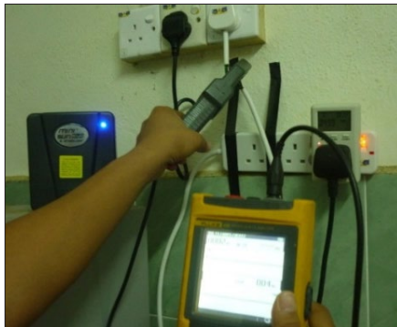
Fig. 7. Recording of data using Fluke Meter
