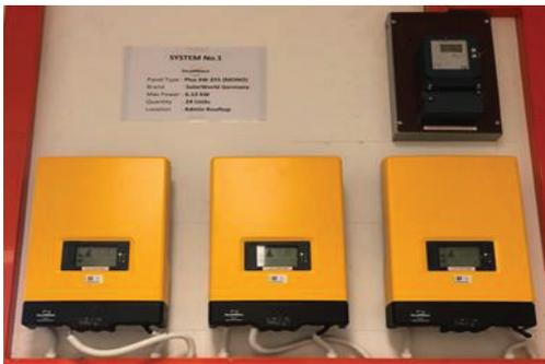
Fig. 2. Installation of 6kW Inverters for monocrystalline PV system at PVSG Lab Weather Station, UTeM
